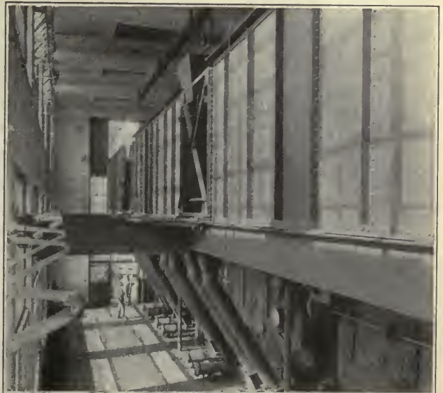
INTERIOR OF BOILER ROOM WITH BUCKET UNLOADING AT MOUTH OF SELF-FEEDING HOPPER
